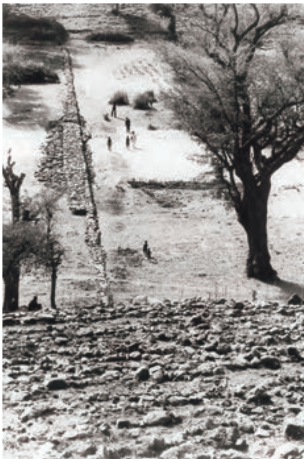
NEF helped communities in Mali's Mopti region build simple stone dams to slow rainwater runoff and improve groundwater recharge, 1988.
